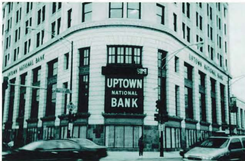
The Uptown Bank building at the corner of Broadway and Lawrence Avenue has been restored.
